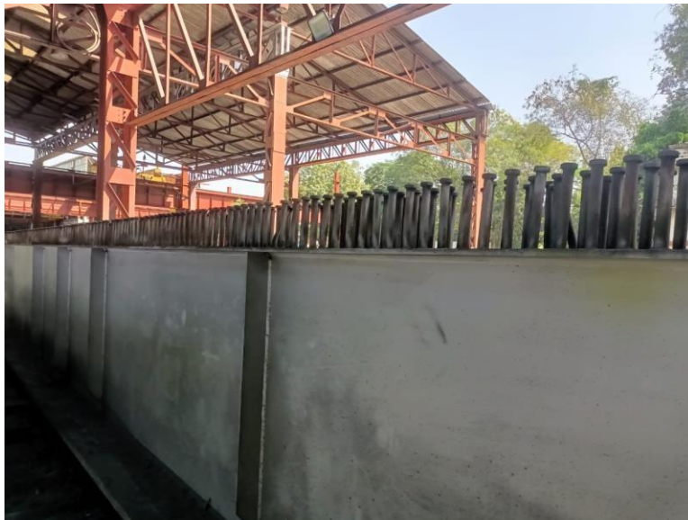
Figure 20: Stud shear connectors
