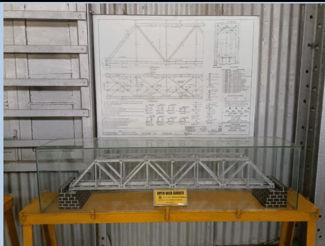
Open Web Girder (61 m Span)
