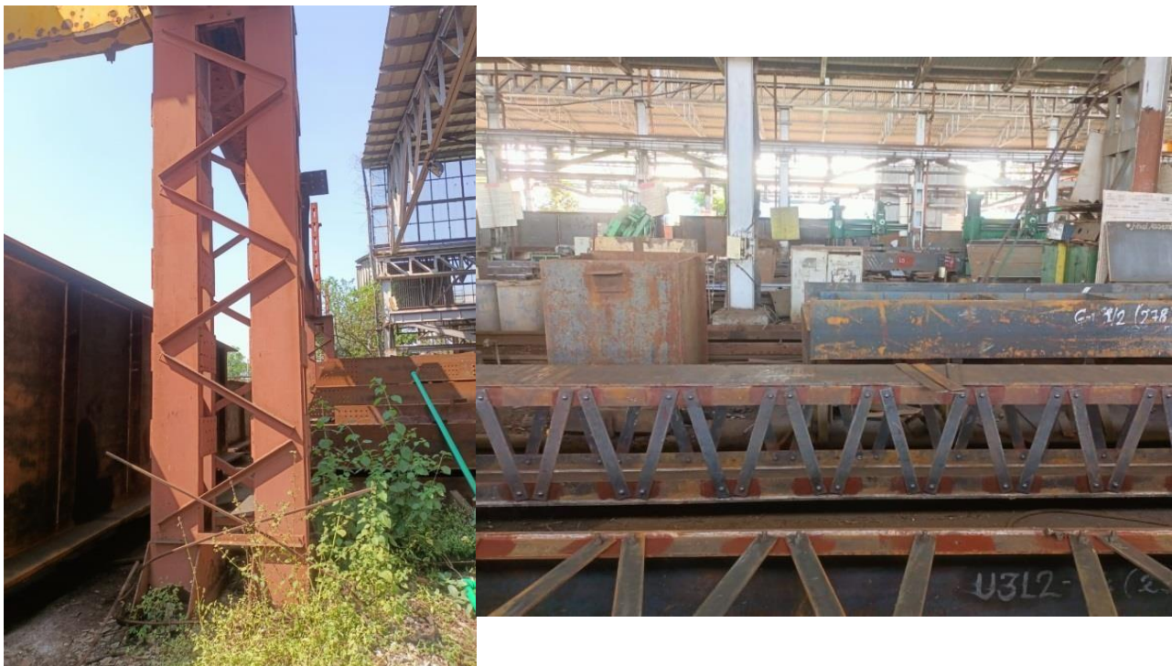
Figure 14: Built-up columns
