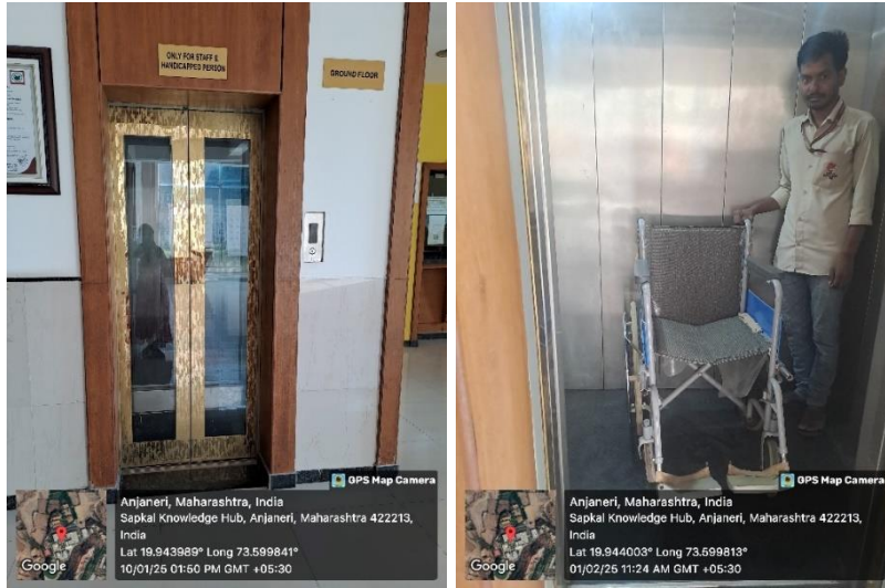
Geotagged photo of Lift and wheelchair provided
