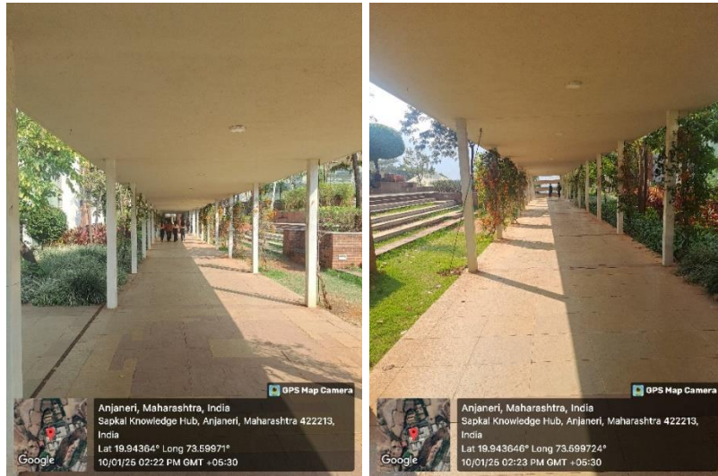
Geotagged photo of covered & broad pedestrian friendly pathways
